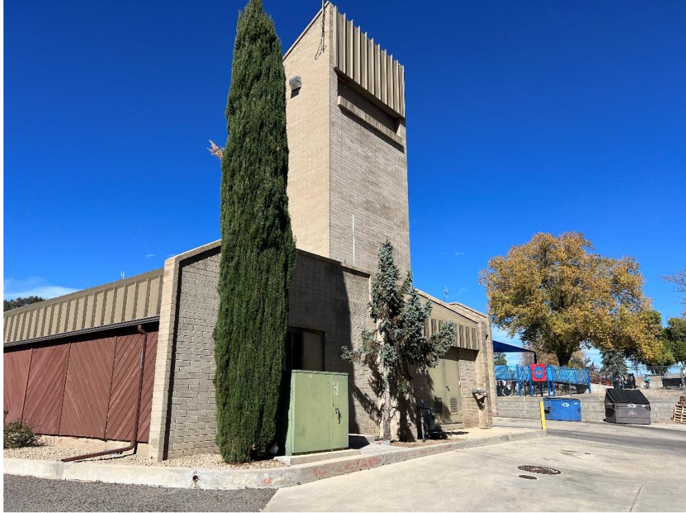
View of hose drying tower.
