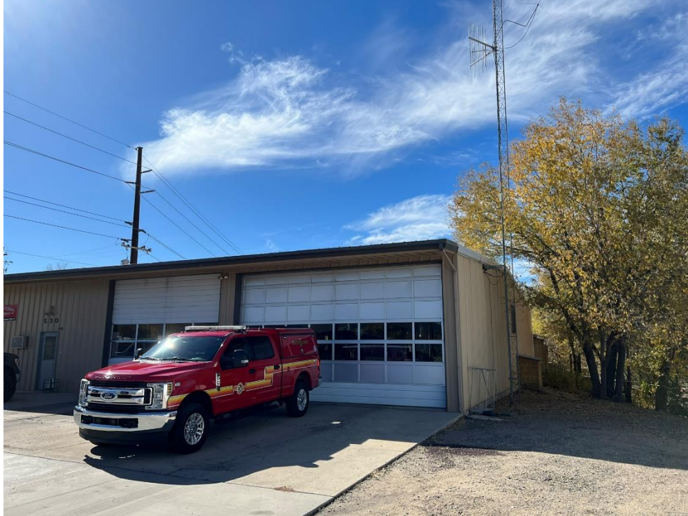
Another view of the front and north side of building.
