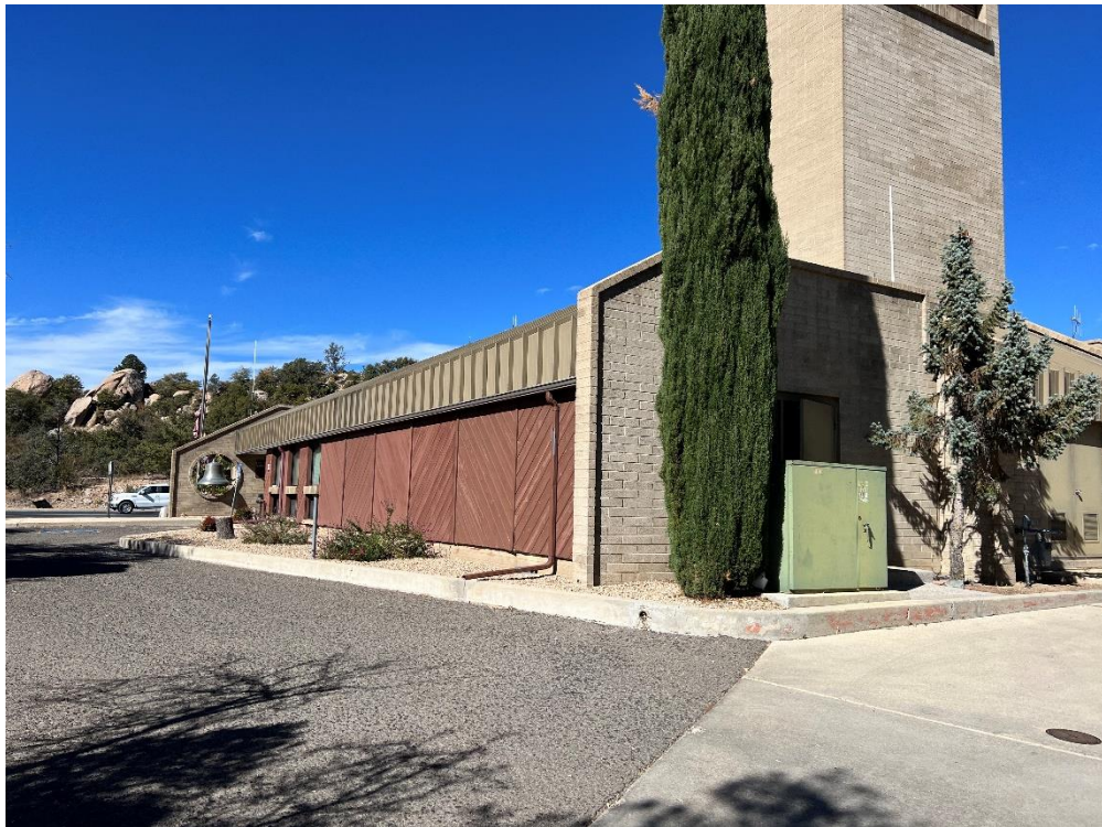
Southeast corner of building looking west.
