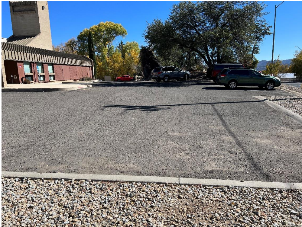
Parking area and south side of building.
