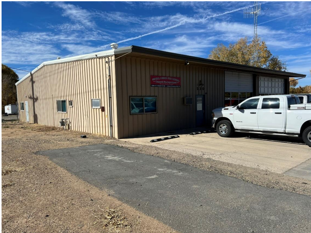
South side of building.
