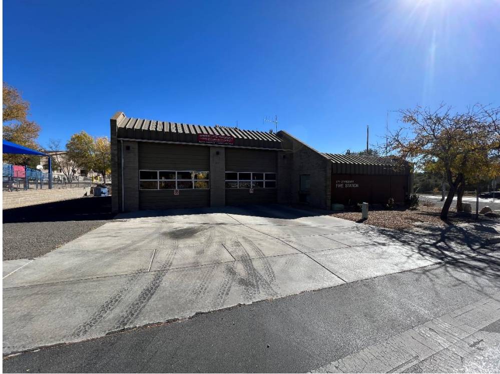
West side of subject from Williamson Valley Road.
