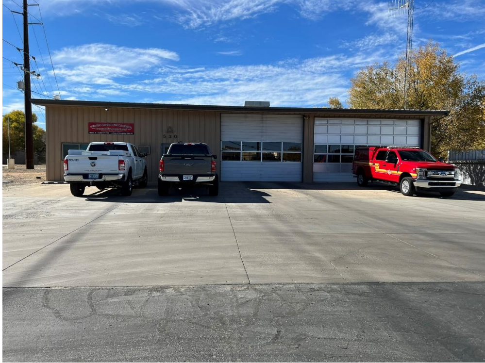
View of front of fire station looking west.
