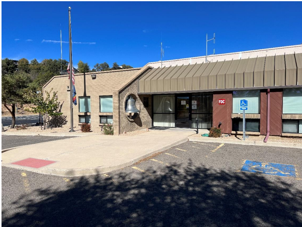
Building entrance on south side.
