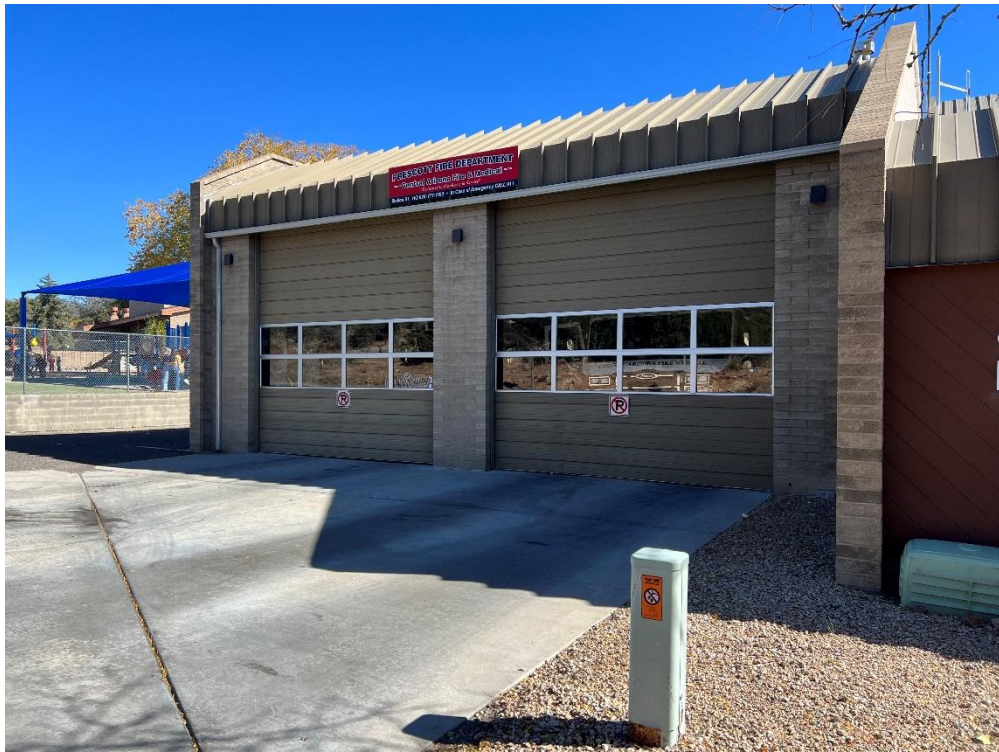
Close-up of truck bay doors.
